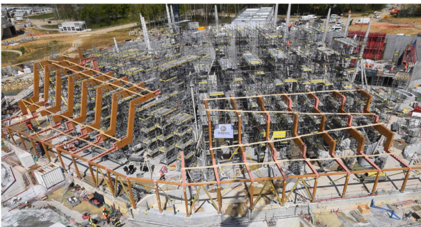
Figure 2: View on construction site
