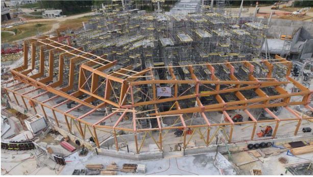
Figure 6: View on construction site
