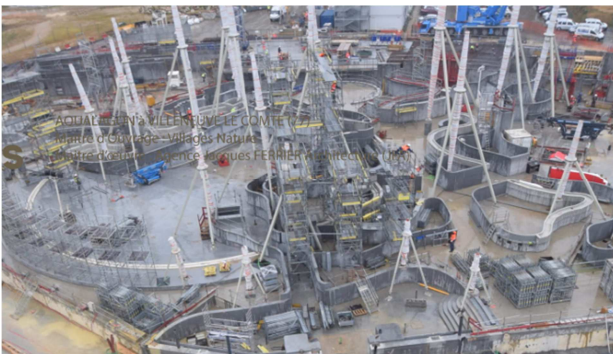
Figure 8: View on construction site: the columns
