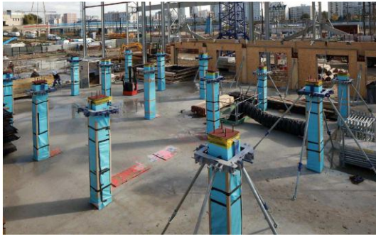
Figure 17: Construction process / Source Arbonis
