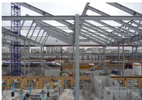
Figure 8: Construction stage wood and steel / JAP Architects
