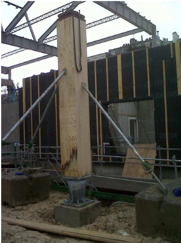
Figure 16: column 400x400 mm / Source Arbonis
