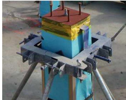
Figure 19: Construction process / post temporary stability / Source Arbonis
