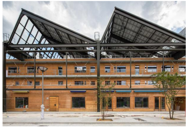
Figure 3: View of the project on Pajol street / Source JAP
