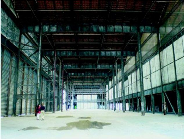
Figure 4: View of the existing building
